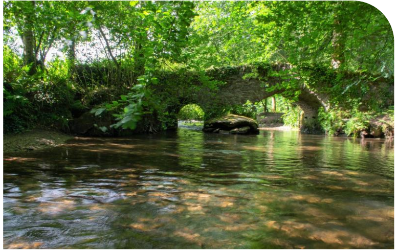
The Grade 2 listed Coldrinnick Bridge
